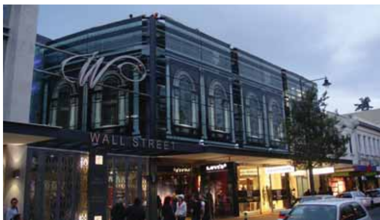
A PRINTED GLASS FRONTAGE WALL ON THE SECOND FLOOR, CLAD TO THE OUTSIDE OF THE BUILDING
